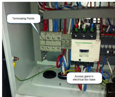
After installation the electrical box should be shut properly to ensure the water ingress rating are maintained. Ensure that the cable is free of hot spots and sharp edges.
