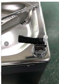
Glass filler installation
