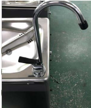
Glass filler installation
