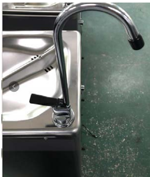
Glass filler installation
